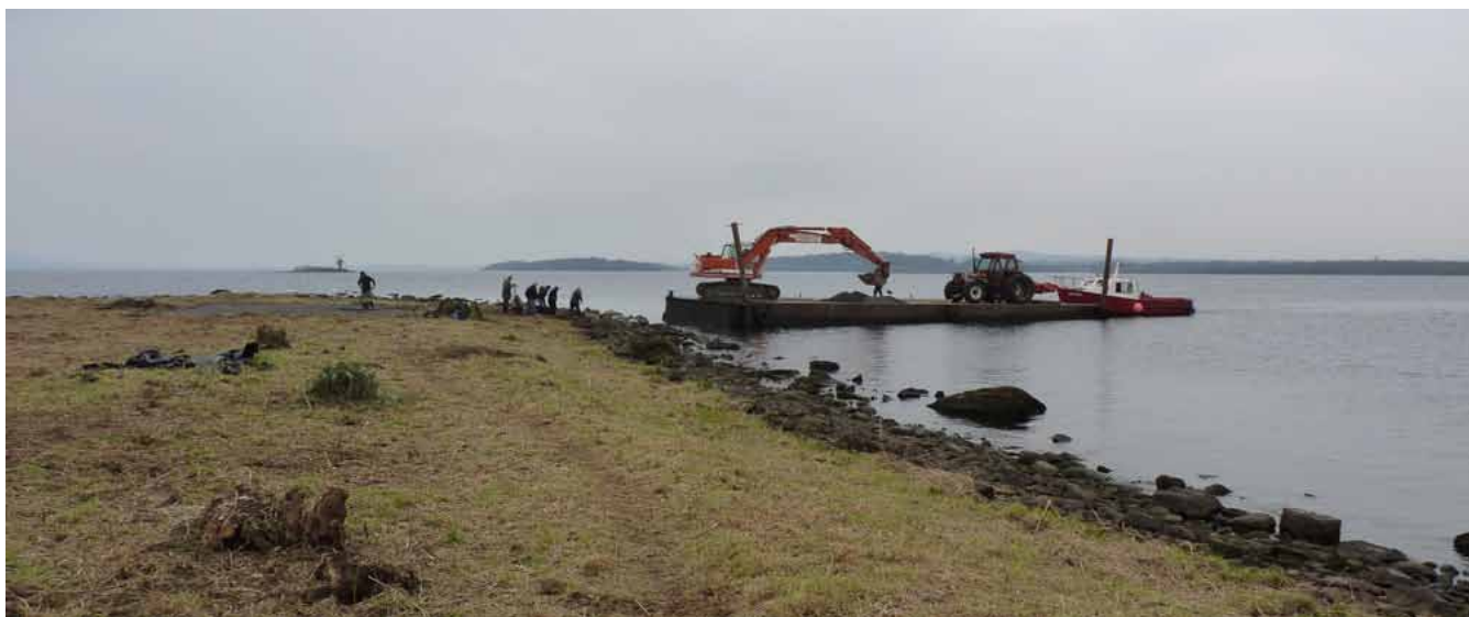
Figure 1 Work to create gravel area on Gravel Ridge Island 2013
